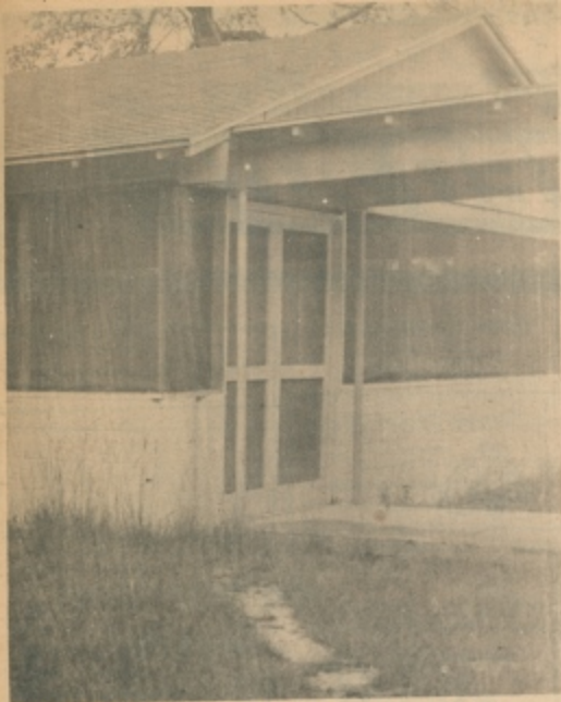
FIRST BAPTIST CHURCH RECREATIONAL BUILDING
