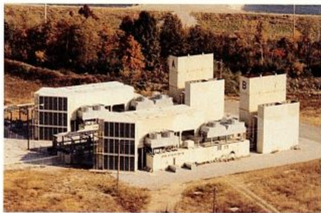
Figure 9. Enclosed two unit ECONOPAC installation
