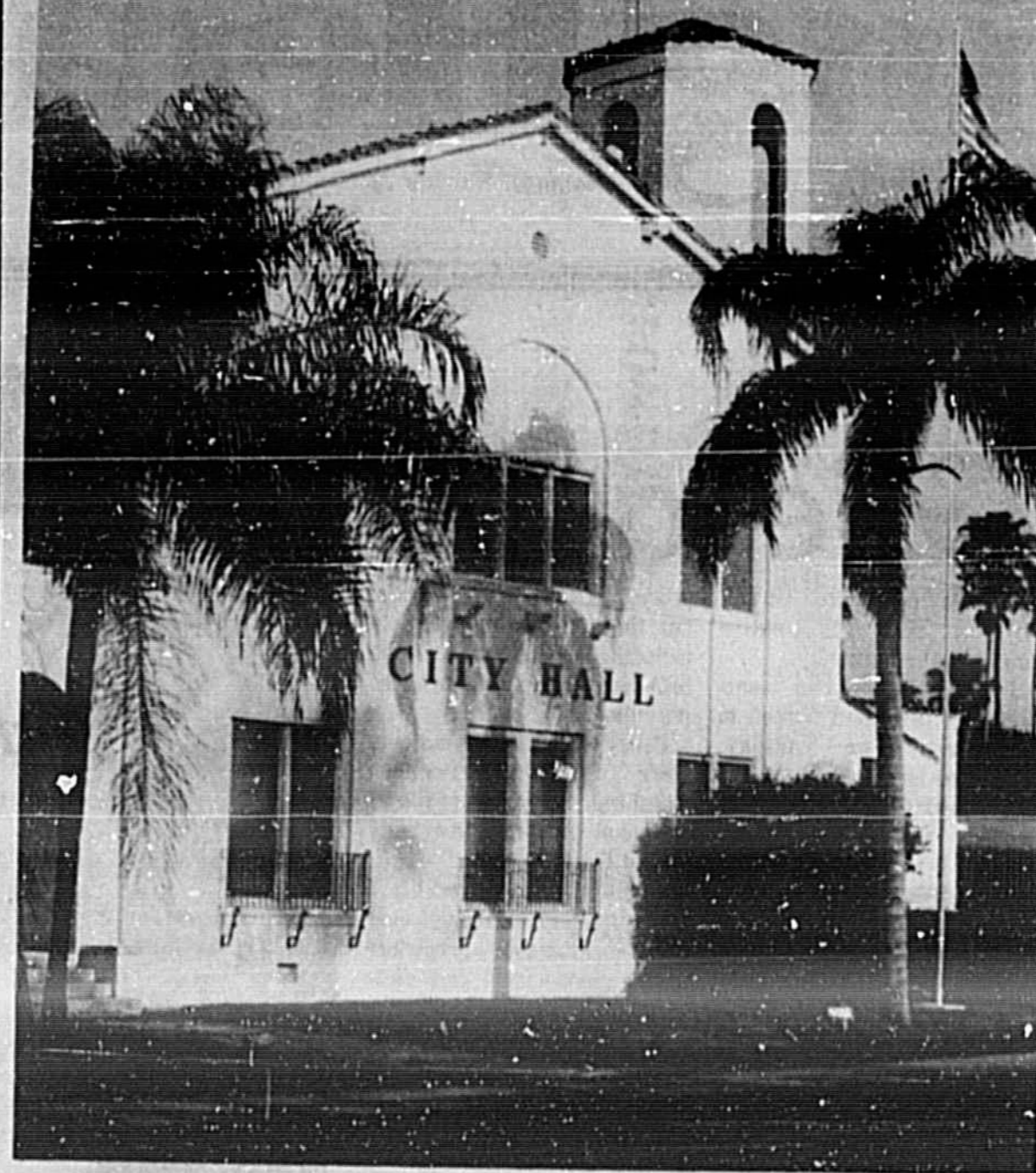
Investigative studies have revealed many defects in Sanford's aging City Hall.
