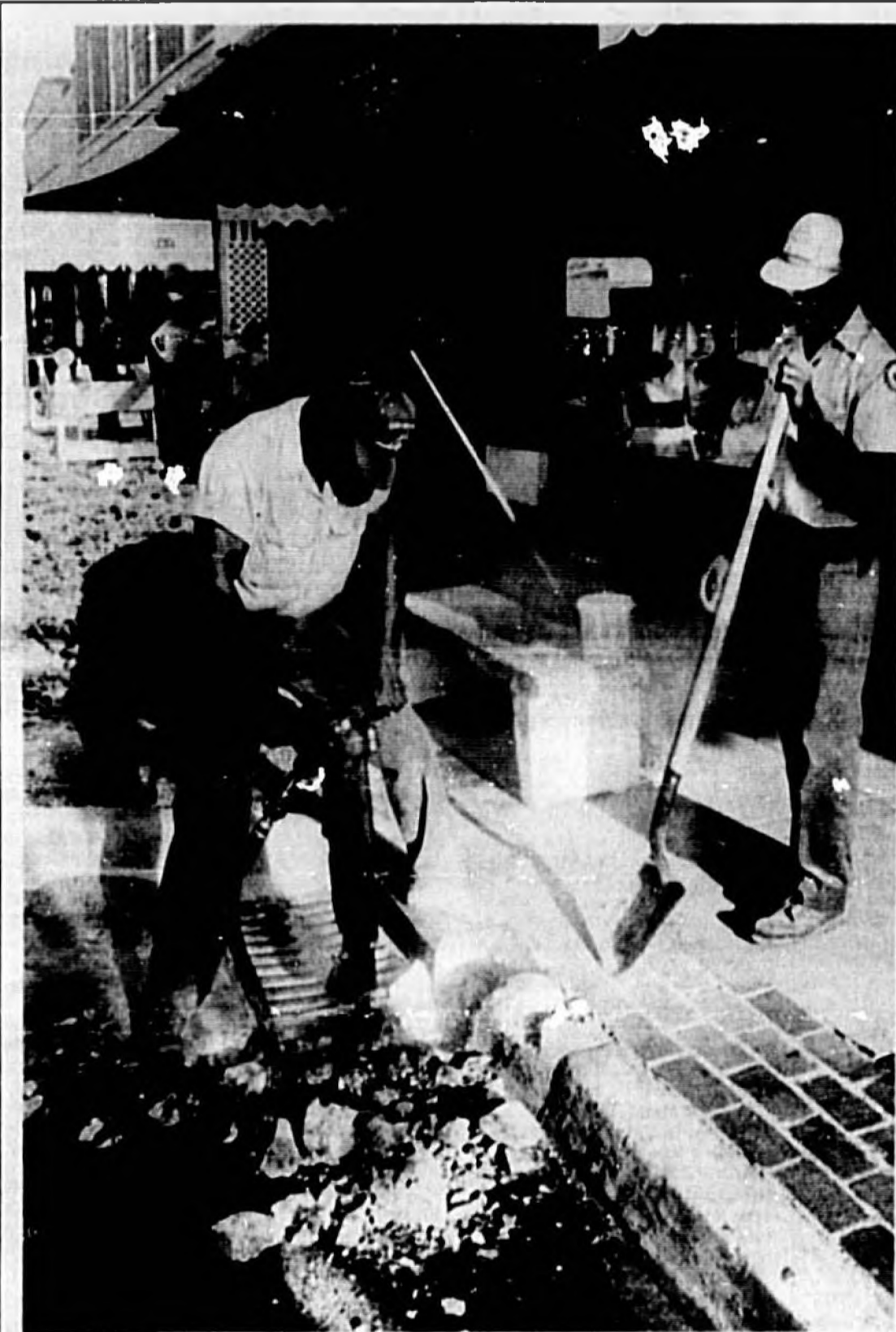
Flood relief work
