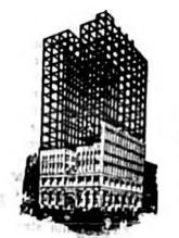
Beneath the beauty of a skyscraper stands a skeleton of steel-hidden, yet holding the greet structure to-
