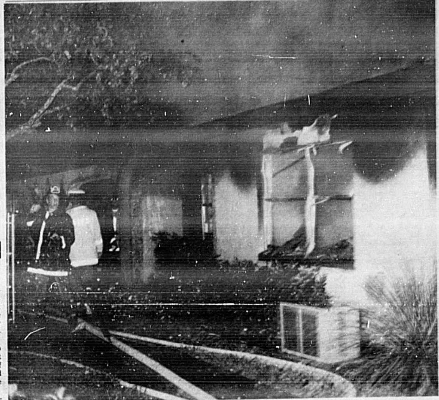
APARTMENT GUTTED BY FIRE Fire from an undetermined origin early today caused an estimated $30,000 loss to a South Seminole apartment; additional furnishings loss was placed at $5,000. Injuries in the blaze that destroyed unit 65 of Sorrento Apartments, located at 2400 Howell Branch Road in Casselberry. (Additional photo page 2A.)
