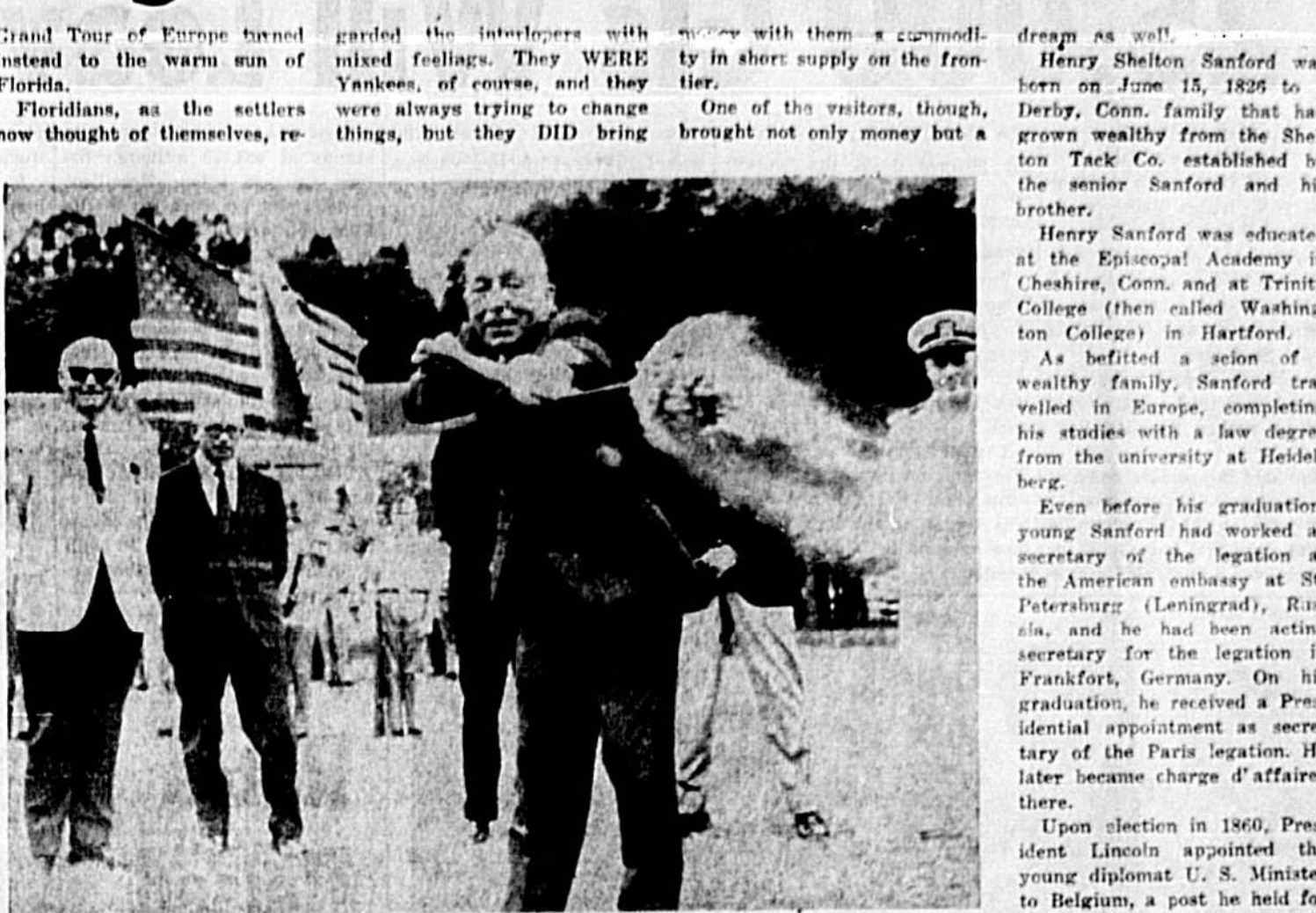
HERE'S LOOKING AT YOU . . . JOSEPH P. WIEGERS, president of the Bernarr Macfadden Foundation, provided a bit of levity at the groundbreaking exercises for the new gymnasium of Sanford Naval Academy, by tossing the first shovel of dirt toward Herald photographer Bill Vincent Jr.
