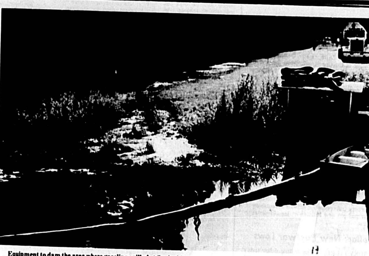
Equipment to dam the area where gasoline spilled at Sanford Port Authority is shown in foreground. The damming is to prevent the gasoline from floating into the canal.
