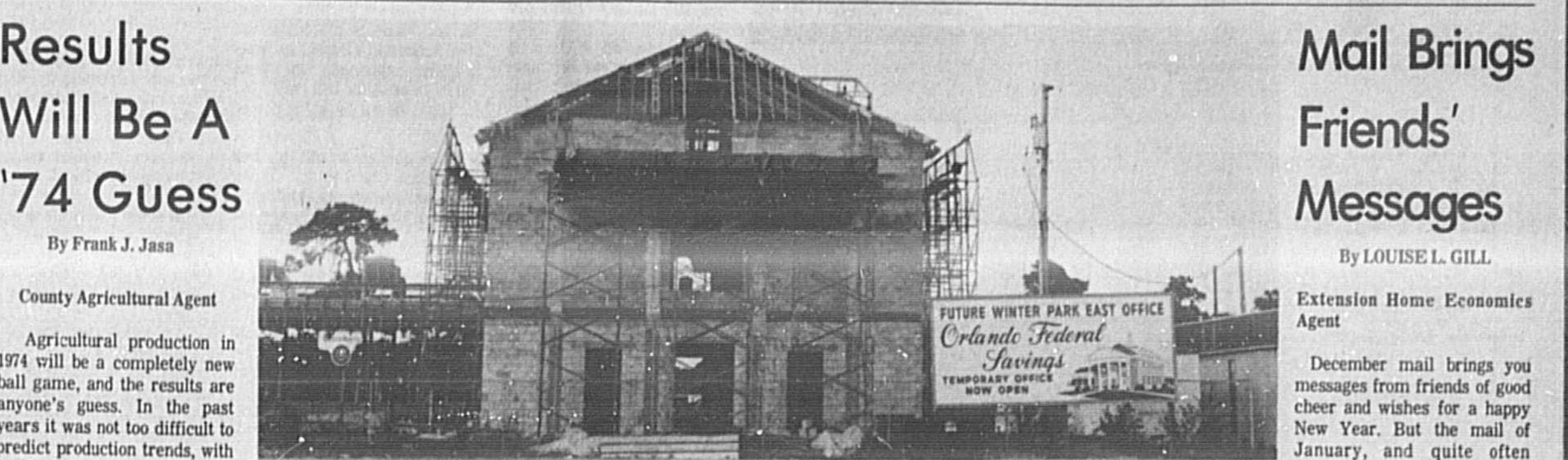
ORLANDO FEDERAL BRANCH UNDER CONSTRUCTION
