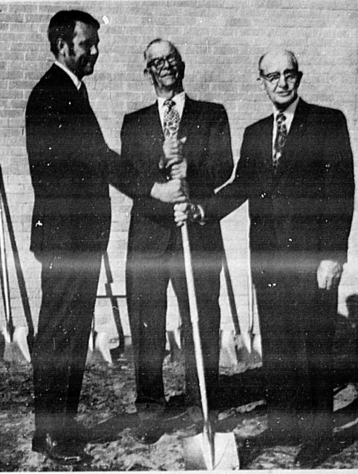
HIGH HOPES Official groundbreaking was held this morning for the new million dollar-plus high-rise addition to First Federal Savings and Loan of Seminole County's First Street facility. Left to right, Gib Edmonds, executive vice president; E. C. Harper Sr., president; and George Touhy, director. (Staff Photo)
