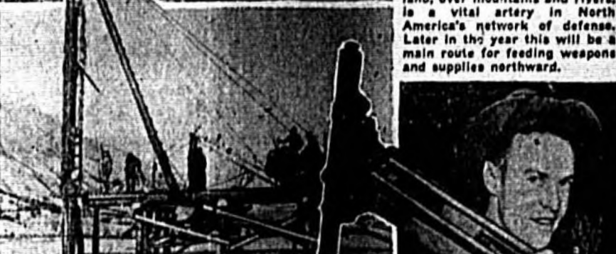
The crash of a pile driver shatters the wilderness silence. Engineers are shown here as they pound bridge supports into a river bed.
