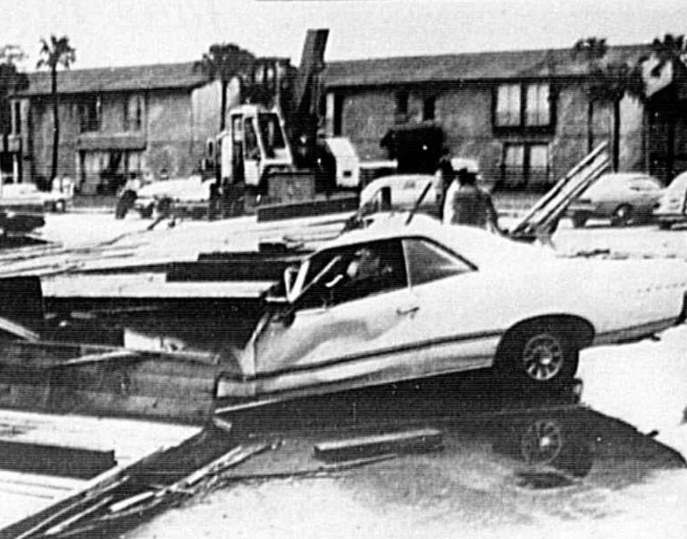
THE ROOF was ripped off eight apartments at the Capistrano Apartments in Altamonte Springs when a tornado hit Tuesday. Altamonte Springs Fire Chief T. L. Siegfried estimated damage at $500,000. Sections of the roof were hurled over the area, crushing cars (above) and falling against other apartments (below). No one was injured.
