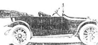
The new light four is a very powerful car, 40 horsepower, and weighs only 2580 pounds. This car is electrically started and lighted by the best system in the world. The body is a perfect stream line design and roomy. The radiator is "V" shaped. The upholstering is comfortable. The seats are wide. The finish is lasting. This car is built
