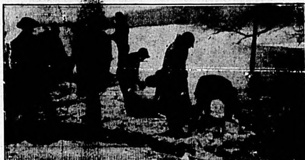
Telling in bitterly cold weather, farmers and boys are shown in a futile fight to check the spread of the flooded Mississippi river in the Bird Point New Madrid floodway by raising the levee near Wolf Island, Mo., with sandbags. It was at the lower point of the floodway that armed farmers prevented government engineers from breaking the levee to relieve Cairo, Ill., of increasing danger. (Associated Press Photo)
