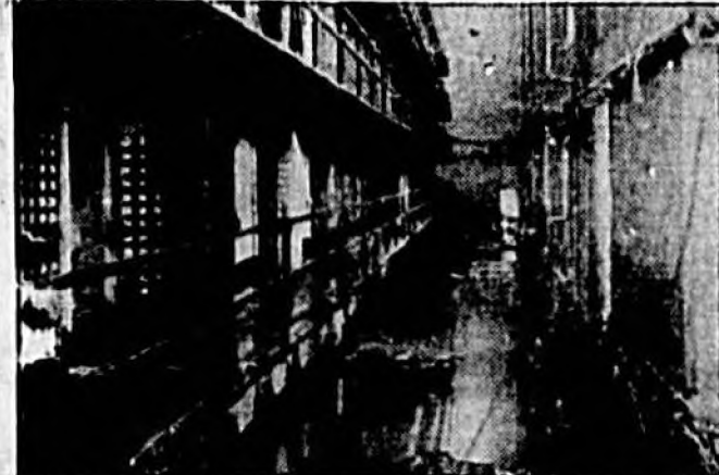
This scene of ruin and wreckage was found in the flooded Kentucky state prison at Frankfort following the evacuation of 3,000 terror-stricken prisoners after three days of panic and wild rioting. No bodies were found, although earlier reports said many had been killed in trying to escape. (Associated Press Photo)
