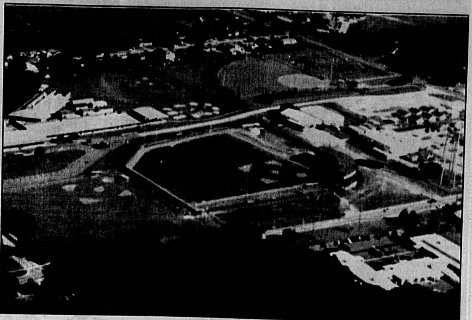
Work will soon begin on Phase III of the renovation project at Sanford Memorial Stadium. The restoration of the stadium, once the spring training home of the New York Giants, is expected to be completed by Spring 2001.
