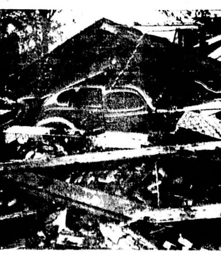
A GARAGE WAS NO PROTECTION for the car as a three-ton roof smashed through Terra Haute, Ind. The walls were blown in and the car crushed in this rubble as the wind tore across the town. Forty-five persons were killed and 100 were injured by the storm which swept the Midwest states.
