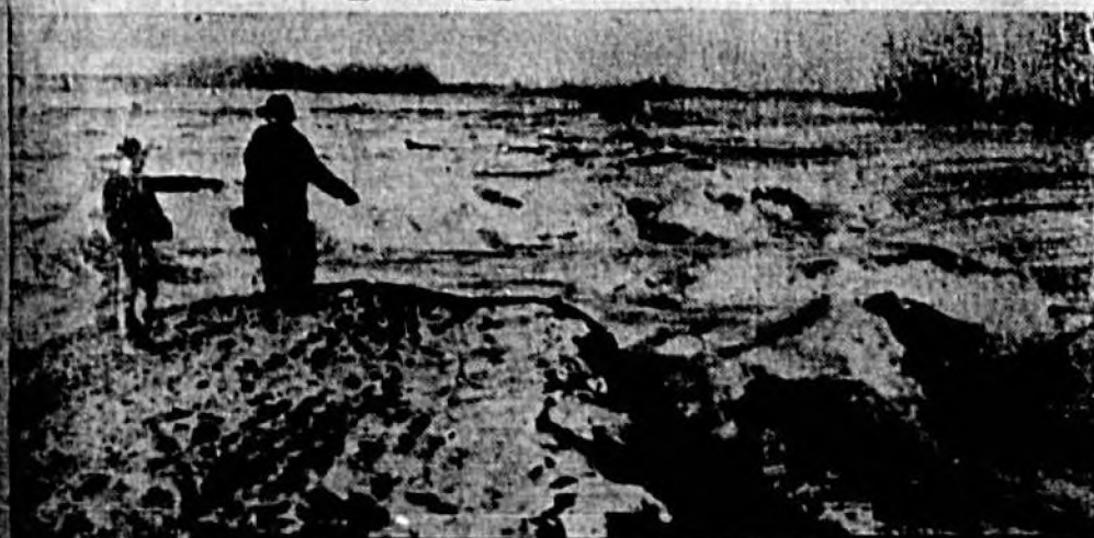
Armed guards with "shoot to kill" orders are patrolling the Redfoot levee near Tiptonville, Tenn., determined to frustrate any attempt to dynamite the dike. It's an old river custom for residents on one side to blow up levees on the other side to release flood water in their own territory. Below, the raging Mississippi is shown rapidly widening the breach in the Beale levee near Tiptonville. When this picture was made the gap was 200 yards wide. (Associated Press Photo)
