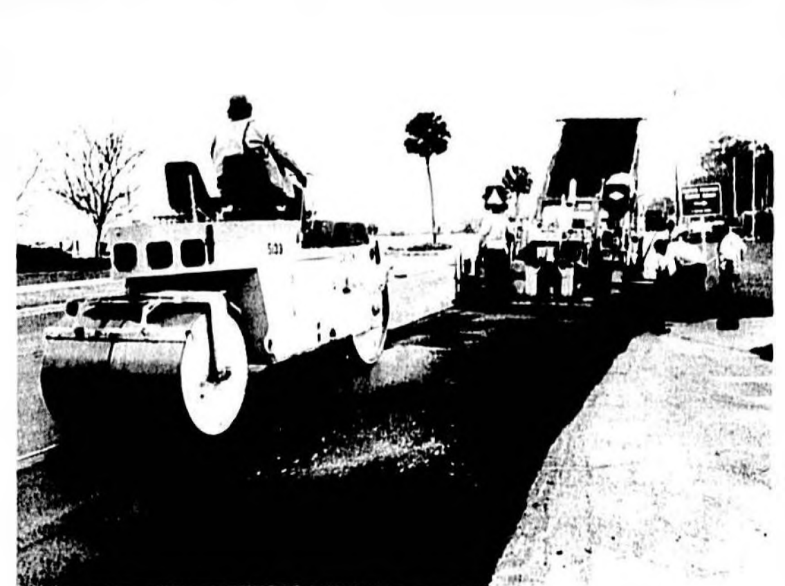
Resurfacing work on a portion of Seminole Boulevard along Sanford's lakefront is expected to be finished by the end of today.
