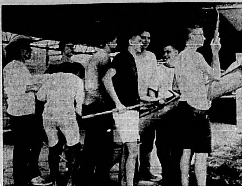
KEY CLUB members at Seminole High School spent Friday afternoon laying a 65-foot sidewalk from the school library to the street. The boys, sponsored by the Kiwanis Club, also bore the cost of the materials from funds they derived from various projects. (Herald Photo)
