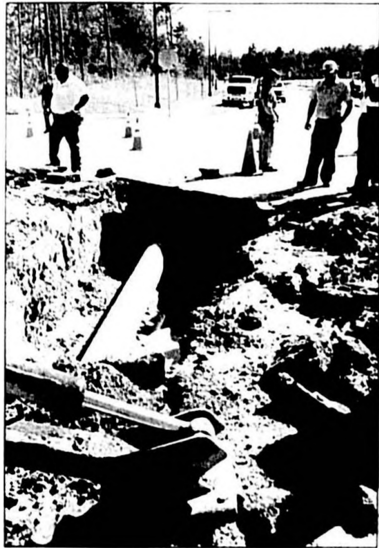
Water from a nearby broken underground pipe caused extensive damage to part of Lake Mary Boulevard Wednesday. Lane closures caused traffic tie-ups between U.S. Highway 17-92 in Sanford and Country Club Road in Lake Mary.
