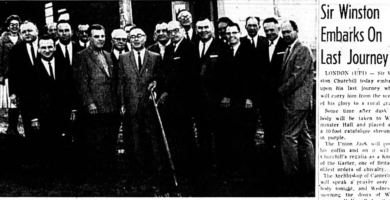
A. B. PETERSON (holding shovel) was given the honor, as chairman of the board of trustees of Seminole Memorial Hospital, of turning the first shovel of dirt this morning, breaking ground for construction of the new $1 million wing. Hospital, city, county and other civic leaders are pictured. (Herald Photo)
