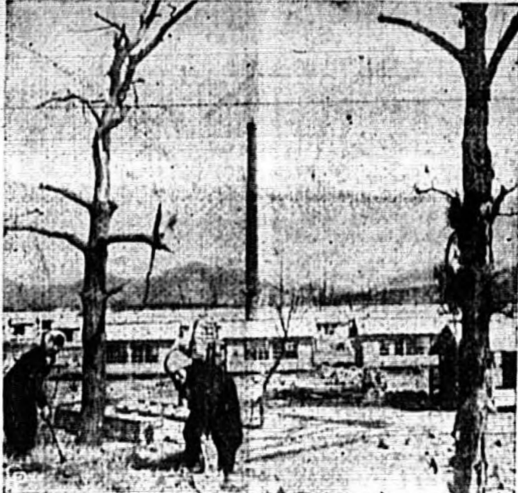
FROM THE RUINS OF JAP WAR FACTORIES obliterated by the atom bomb seven months ago rises a housing project to provide shelter for the citizens of the stricken city of Hiroshima. The one-story homes are neatly lined up on plots cleared of rubble. Lifeless trees, killed by the mighty atom blast, are shown in the foreground. (International)
