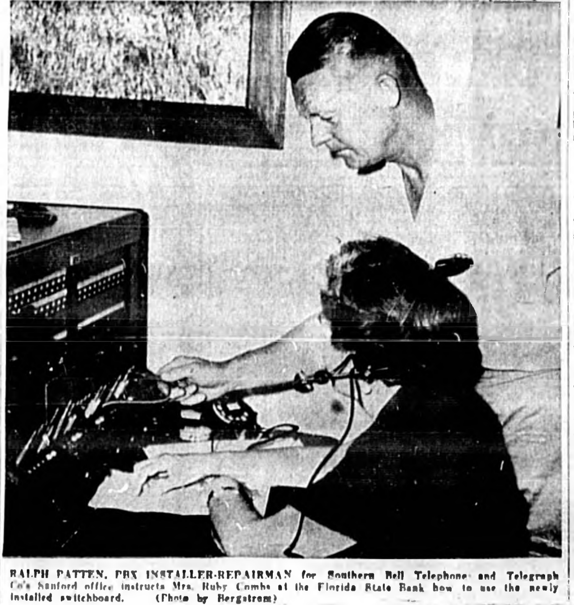
RALPH PATTEN, PBX INSTALLER-REPAIRMAN for Southern Bell Telephone and Telegraph Co.'s Sanford office instructs Mrs. Ruby Combs of the Florida State Bank how to use the newly installed switchboard. (Photo by Bergstrom)
