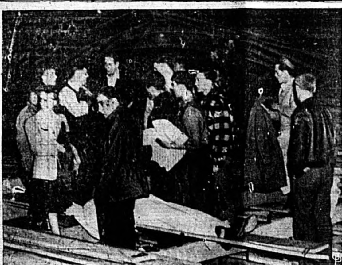
WHERE 250 WERE INJURED in University Stand Collapse. Spectators stand amid the wreck- age of the wooden stands that collapsed in Pu rdoe University. Fieldhouse was sealed until officials open an investigation into the accident.
