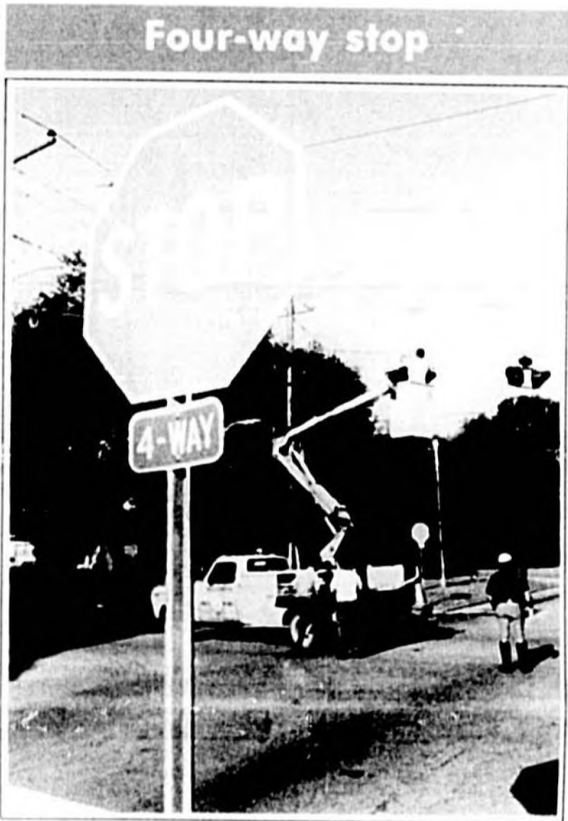
The Public Works Department installs a red flashing light (background) at the intersection of Mellonville Avenue and 20th Street Monday to convert the intersection into a four way stop. Previously a two way stop, the intersection has been the scene of numerous accidents over the years, prompting the change.
