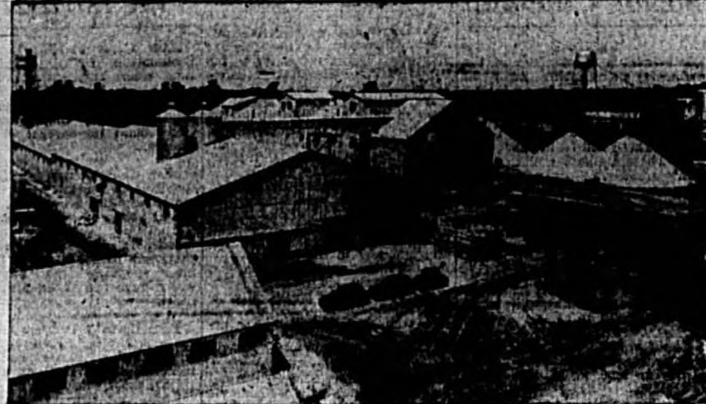
NEW $1,500,000 National Gypsum plant which was formally opened May 22nd at Savannah, Georgia, has an annual capacity of 125,000 tons of gypsum product and will manufacture plaster, plaster wallboard, gypsum lath and sheathing. The Savannah unit will serve the entire southeast with a full line of gypsum products.
