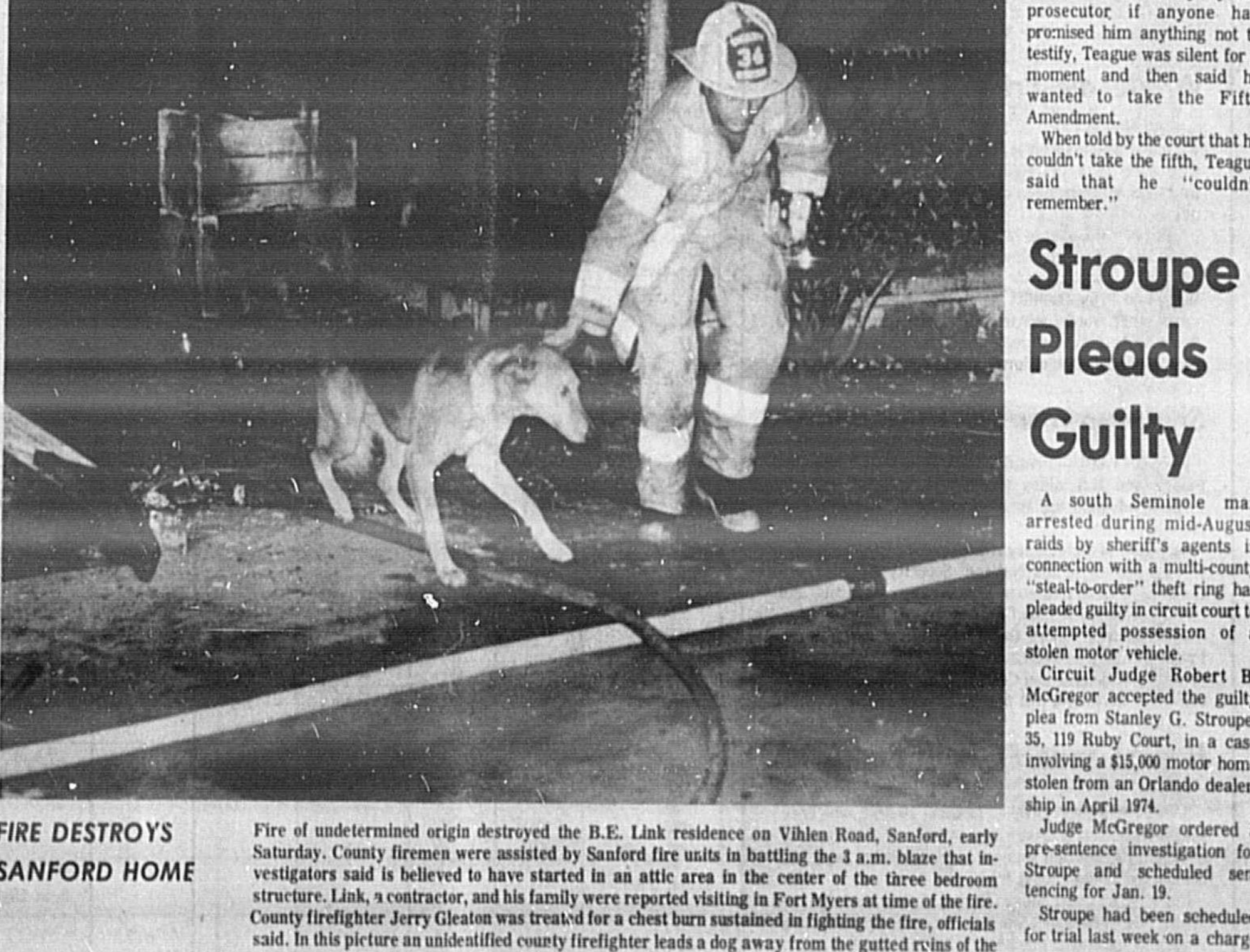
FIRE DESTROYS SANFORD HOME Fire of undetermined origin destroyed the B.E. Link residence on Viblen Road, Sanford, early Saturday. County firemen were assisted by Sanford fire units in battling the 3 a.m. blaze that investigators said is believed to have started in an attic area in the center of the three bedroom structure. Link, a contractor, and his family were reported visiting in Fort Myers at time of the fire. County firefighter Jerry Gleason was treated for a chest burn sustained in fighting the fire, officials said. In this picture an unaffiliated county firefighter leads a dog away from the gutted ruins of the structure. (Herald Photo by Tom Vincent)
