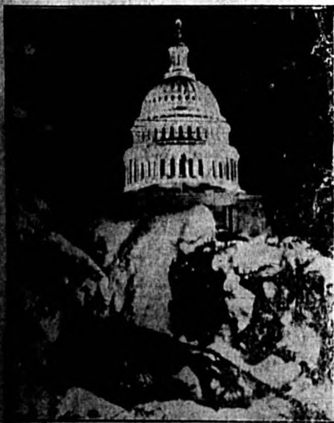
Snow drifts and evergreens formed a natural frame for this night picture of the Capitol as Washington dug its way out of heaviest snowfall in 14 years. (Associated Press Photo)
