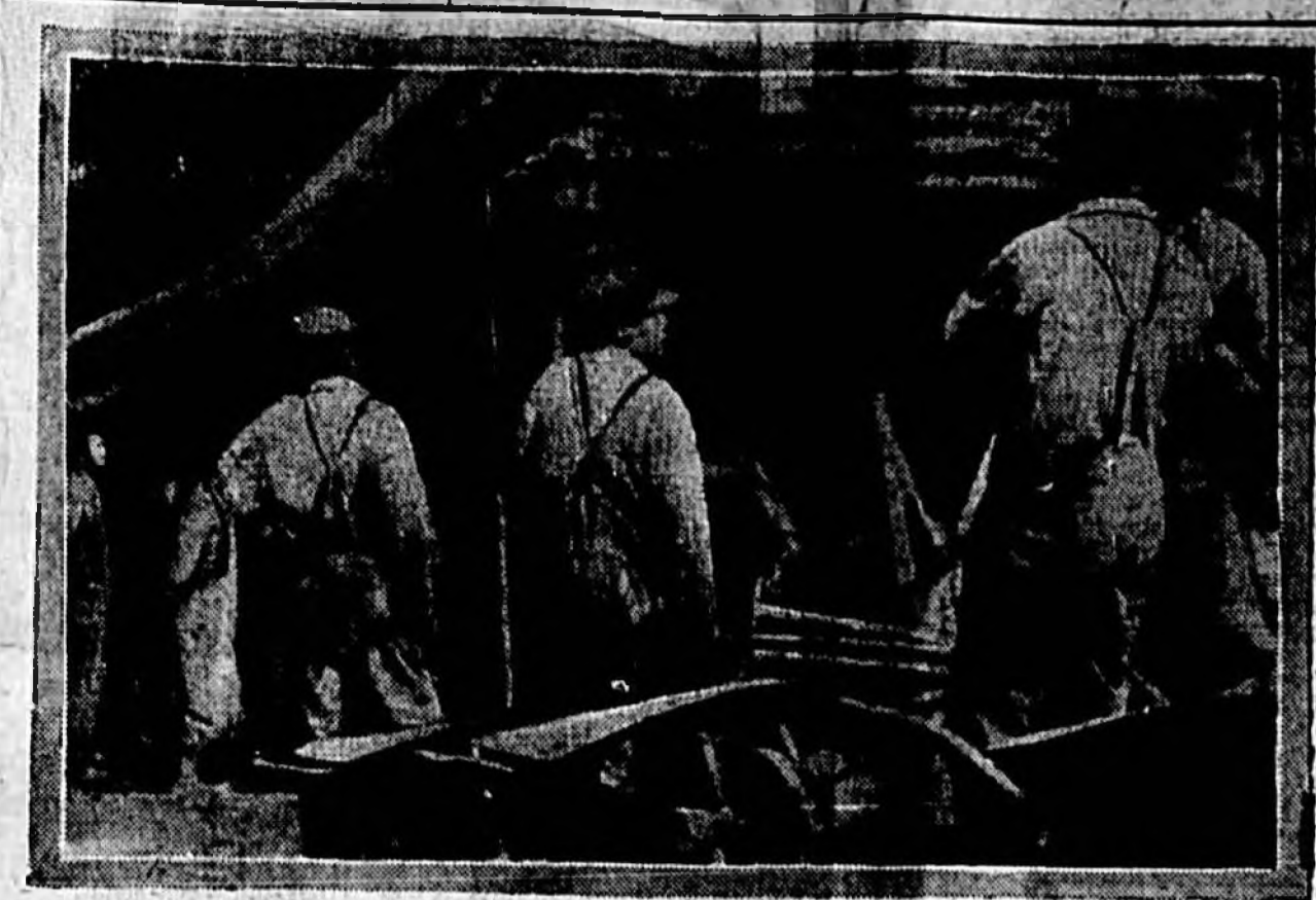
This picture was taken at the mouth of the shaft dug to reach Floyd Collins at San Cave, Kentucky, just as workers were changing shifts. The rope shown in the center of the photo was used to haul stone and shale to the surface.
