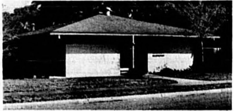
Dr. William Runge's Park Avenue office is identified by on the face of the building. But Runge says he needs a sign in the yard so the office can be identified from the road. on zoning because the court deemed Sanford had granted too many variances. The new city commission's position has been that variances weaken the law. Under multi-family zoning, signs are not allowed on professional offices.
