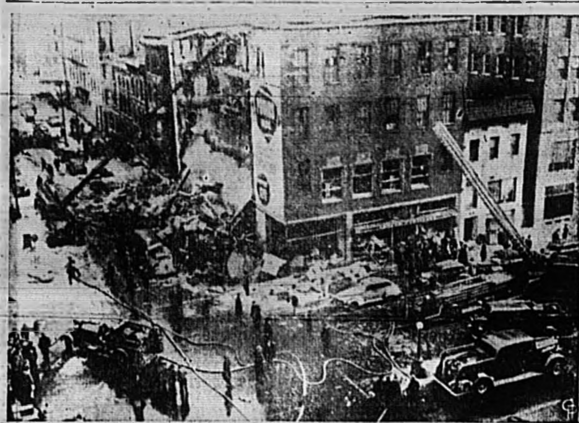
FIVE PERSONS WERE KILLED and six injured when an explosion blew out a complete wall of this four-story furniture building in Chicago. The blast occurred shortly after a company employee reported a gas leak. Cars parked near the wrecked structure were damaged by pieces of household articles. (International)
