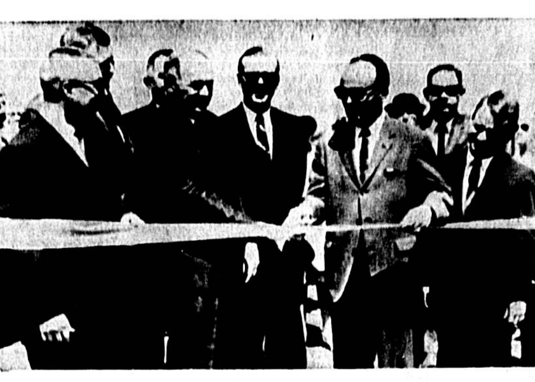
JAY BROWN and G. A. Bennet, state road commissioner and district engineer, respectively, cut the ribbon as dignitaries look on this morning when the Lake Mary interchange of Interstate 4 was opened to traffic. (Herald Photo)
