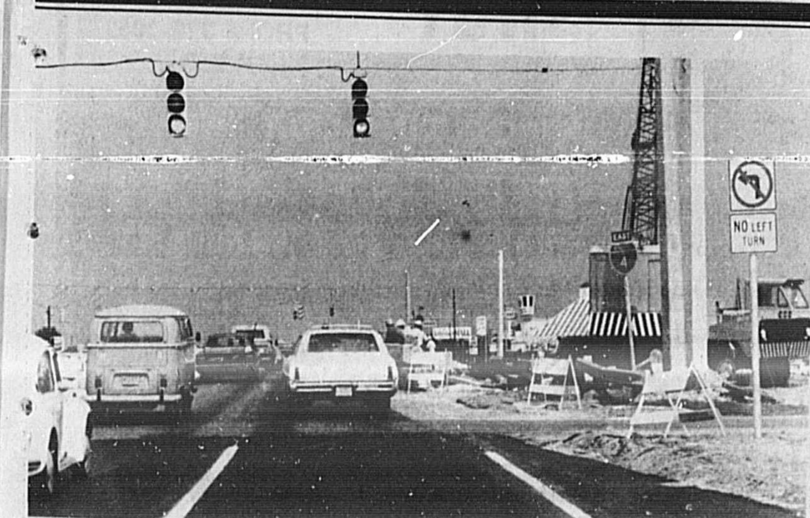
ALTAMONTE'S TRAFFIC JAMMED Revamping of the SR 436 bridge over Interstate I-4 in Altamonte Springs from four lanes to seven much traveled intersection. Completion of the job, tied in with other area road improvements, however, is expected to take 12 more months. Rather than two lanes in either direction, the revamped bridge will also have two left turn Westbound lanes onto I-4 and one left turn eastbound lane to I-4. A traffic count by the state Department of Transportation prior to the opening of the Altamonte Mall last summer at the I-4-SR 436 spot showed 35,000 vehicles per day going through the intersection.
