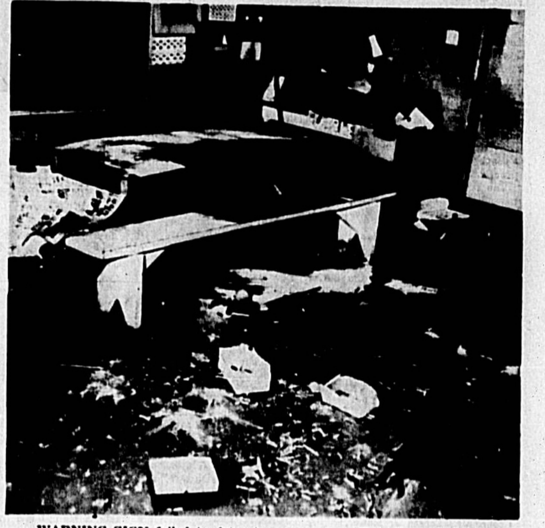
WARNING SIGN failed to deter two young boys Saturday and Sunday and they smashed their way through Pinecrest School, leaving wake of destruction in rampage through school's 38 rooms. Alarm system installation had not been completed, although signs were posted. (Herald Photo)
