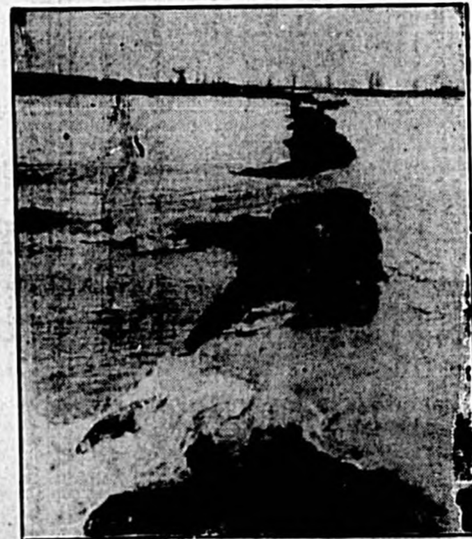
The first setback encountered by engineers in their dramatic battle to hold the flooded Mississippi within bounds occurred near Boss Landing, Tenn., when the torrents broke through a secondary levee in two places, inundating about 20,000 acres. Water is shown cascading through the gaps. (Associated Press Photo)
