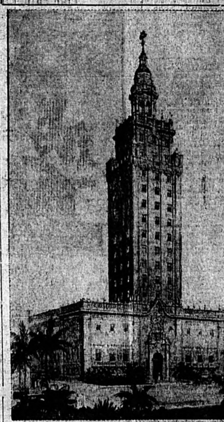
This is the News Tower building of Miami, Florida, now being constructed for the Miami Daily News...
