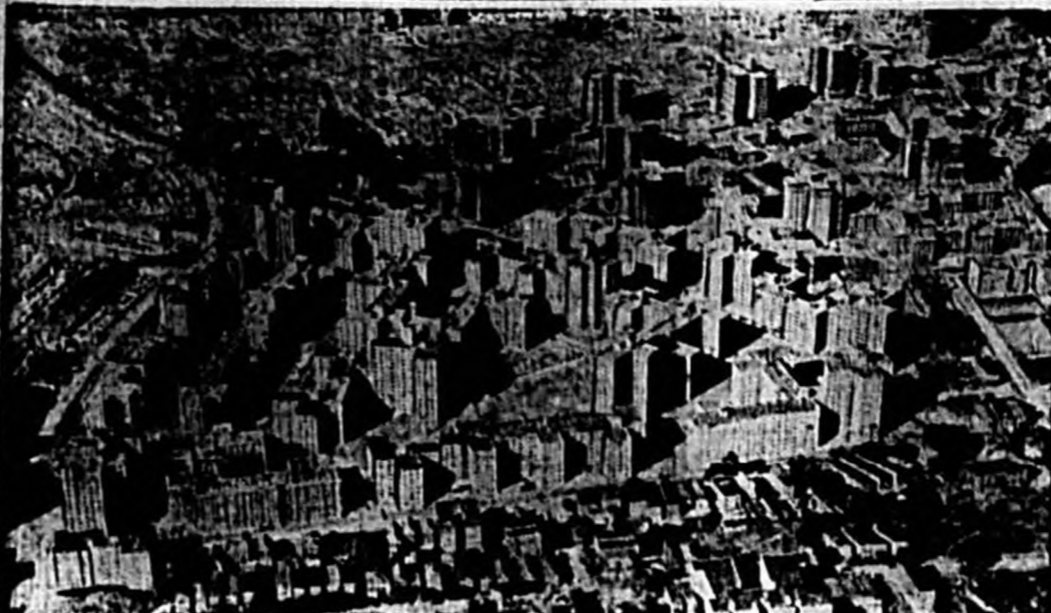
Striking airview above shows construction partially completed on Parkchester, the City Within a City being built in New York's borough of the Bronx. When finished, Parkchester's 51 buildings, containing 12,273 apartments, which will rent at about $13 per room per month, will have cost their owner, the Metropolitan Life Insurance Company, close to $50,000,000.
