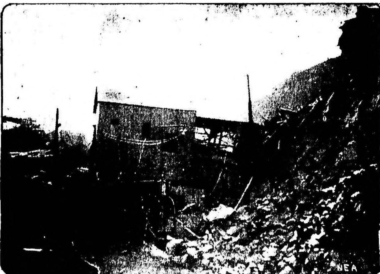
A strip of land half a block wide and a block and a half long in the heart of the Memphis (Tenn.) river front business section sank 50 feet after the Mississippi river had subsided at its base. This photo shows what it looked like afterward. Notice that the electric light poles are still upright, while at the upper right may be seen the "bluffs" left by the ground's recession.
