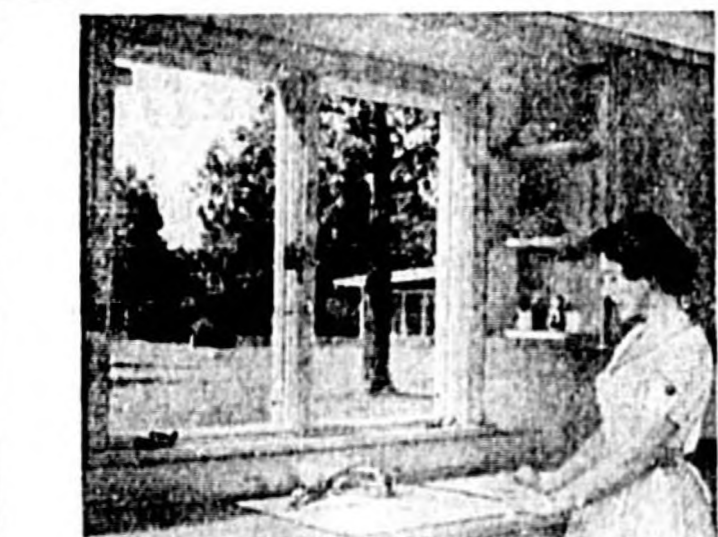
WINDOWS ARE IMPORTANT in modernizing a kitchen. Plenty of light is essential; good ventilation is, too. Windows should open and close readily. Even a short person should be able to handle them easily leaning over a sink or countertop.
