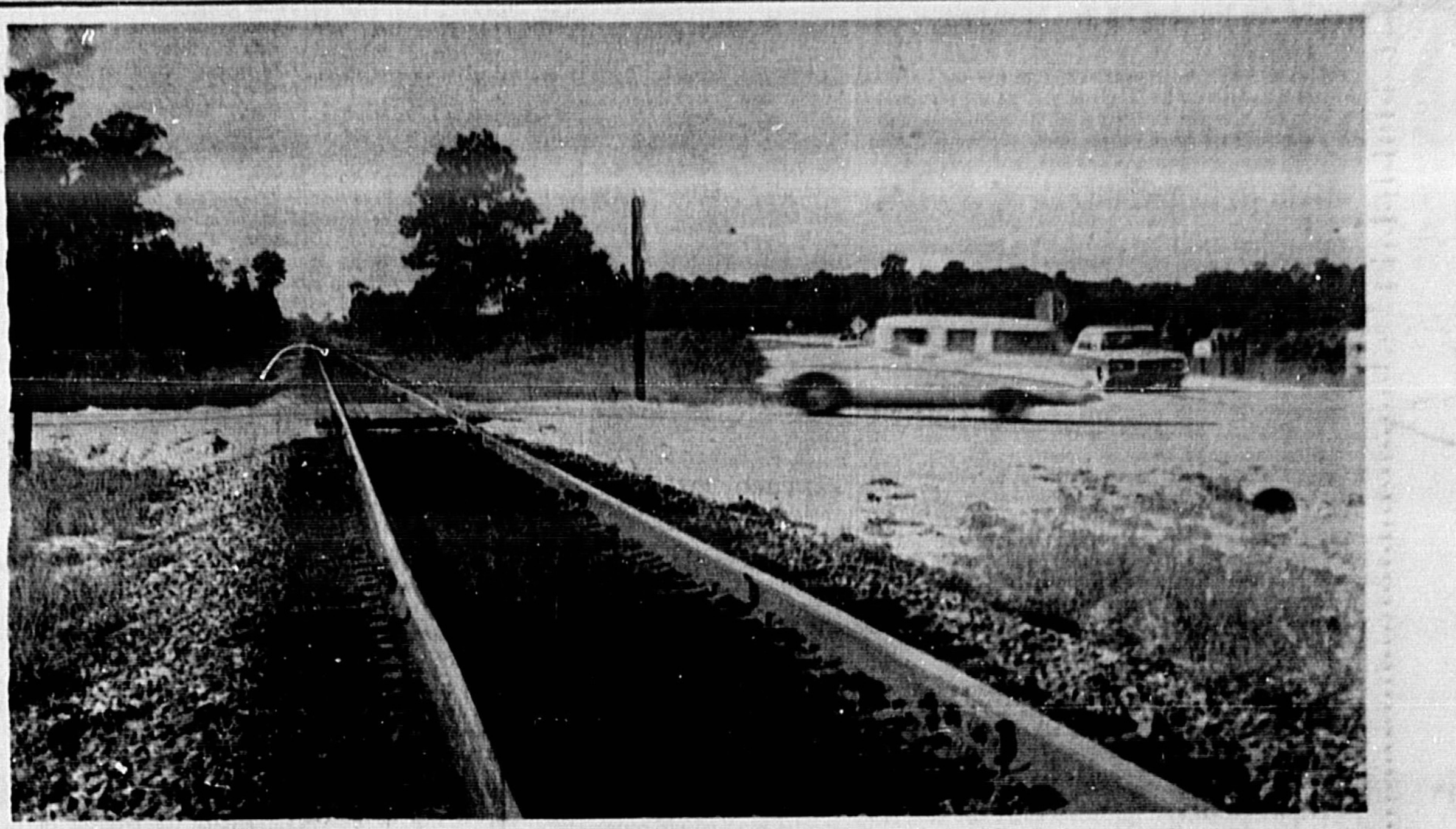
NOTHING ON THE TRACK... THIS TIME! A delegation of Seminole County is the newly constructed Onora Road extension where it crosses Lake Mary Boulevard. Formerly a four-way stop, autos traveling on Onora Road now have the right-of-way, permitting blurs-of-action to whiz across the railroad. (Bill Vincent Photo)
