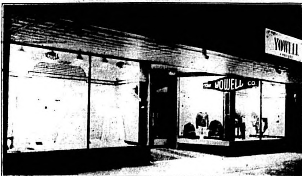
Yowell's, the only department store in Central Florida which boasts air conditioning, has been thoroughly remodeled inside and out at a cost of between $15,000 and $20,000, and is one of the most up-to-date and attractive stores to be found between Jacksonville and Tampa.
