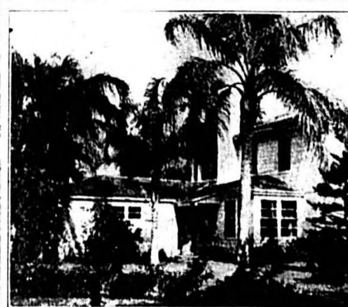
Among the most beautiful homes of Central Florida recently completed is that of Edmund B. Stowe, located at Indian Mound Village, overlooking the St. John's River. The residence is of partial masonry and frame construction with a single tile roof. It is insulated with rock wool and concrete and terrazzo floor, lined with a copper termite shield, insulating against the ravages of termites and the attacks of insects.
