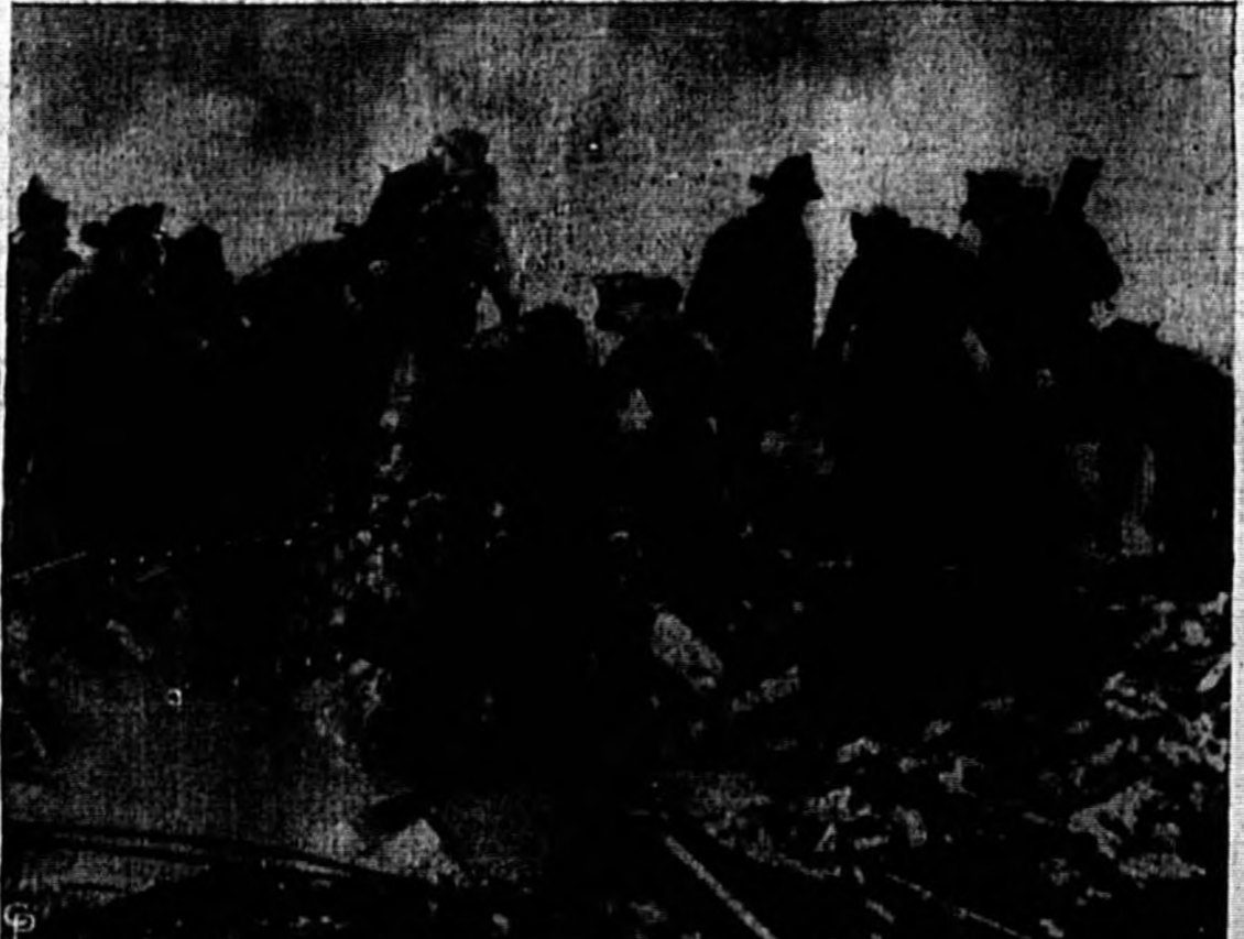
FIREMEN ARE SHOWN hunting through the debris for victims of the blast in the Chicago Loop area which demolished a 3-story building and badly damaged nearby elevated tracks and buildings. At least three were known to be dead and 46 injured. The terrific explosion was near the La Salle Street railroad station in the heart of the heavily populated wholesale district. Had it occurred on a week-day the life toll would have been terrific, say officials. (International)
