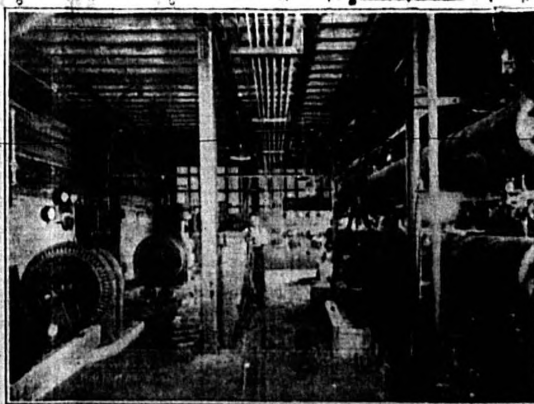
VIEW OF ENGINE ROOM
