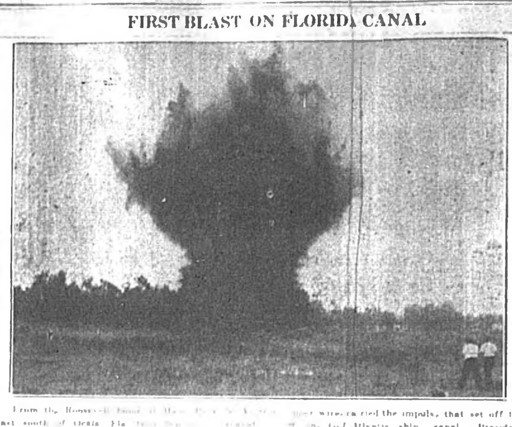
FIRST BLAST ON FLORIDA CANAL
