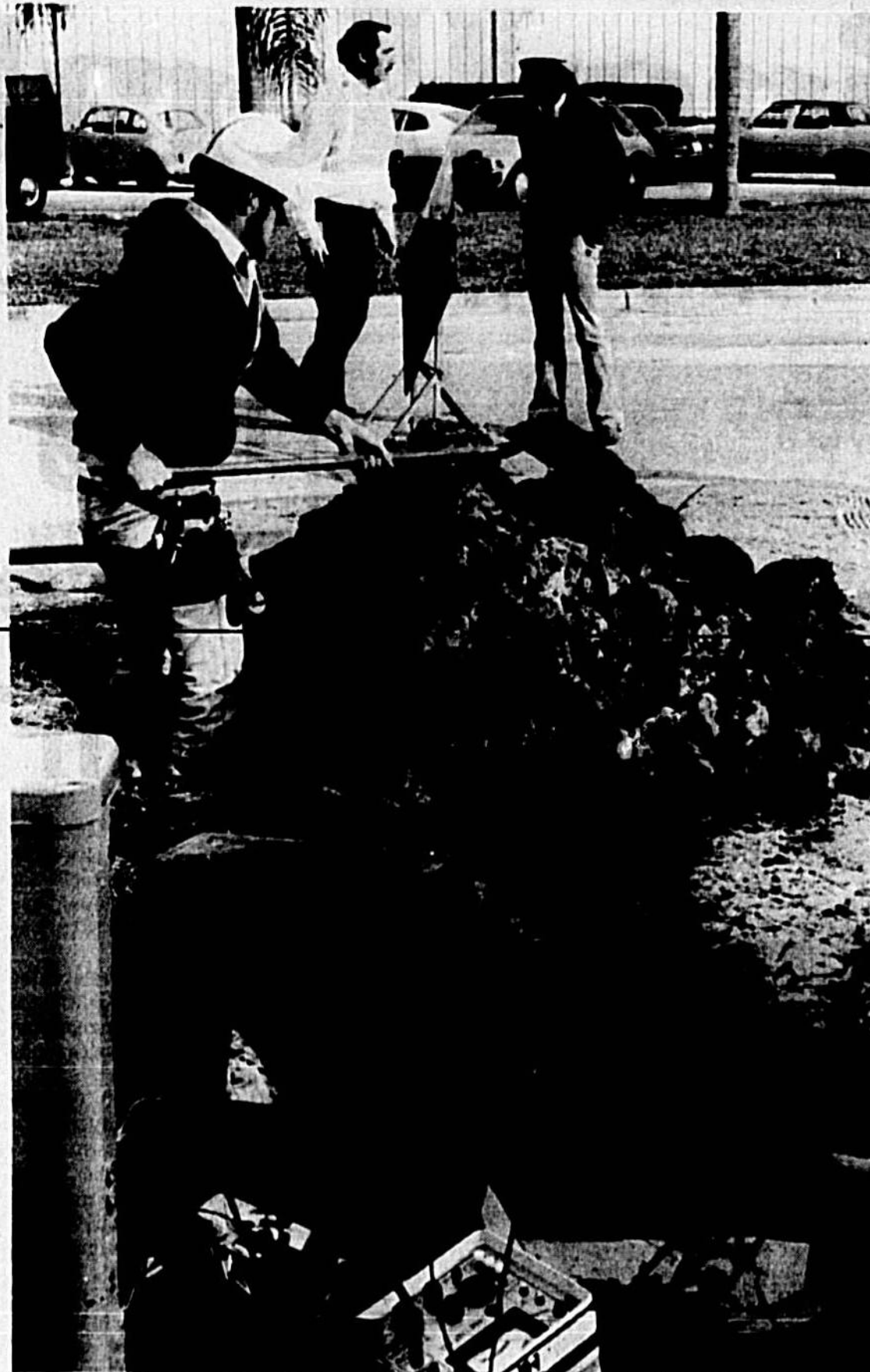
Southern Bell repairman Tom Livingston digs around cable while, in background, supervisor David Maxwell discusses situation with Charlie Jensen of the Sanford engineering department.
