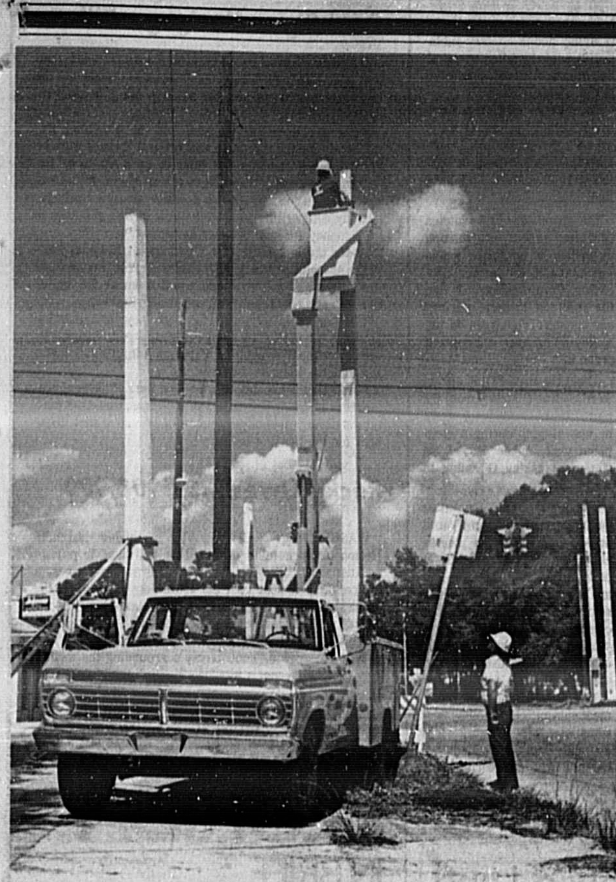
City of Sanford crew moves concrete utility pole at 25th Street and Sanford Avenue after state Department of Transportation installed new pole, left, moving traffic signal supports further from intersection. Wooden pole in center was temporarily installed by city to facilitate modification work.
