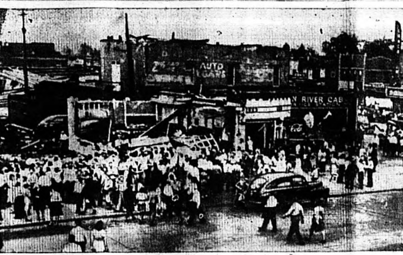
Crowds mill about in the business section of River Rouge on the outskirts of Detroit after a tornado struck the city by surprise, killing seventeen persons and injuring over 200 others. At right, a motion picture theatre stands badly damaged while in the foreground a crowd has gathered about a service station that has been completely ripped apart by the fury of freak storm.
