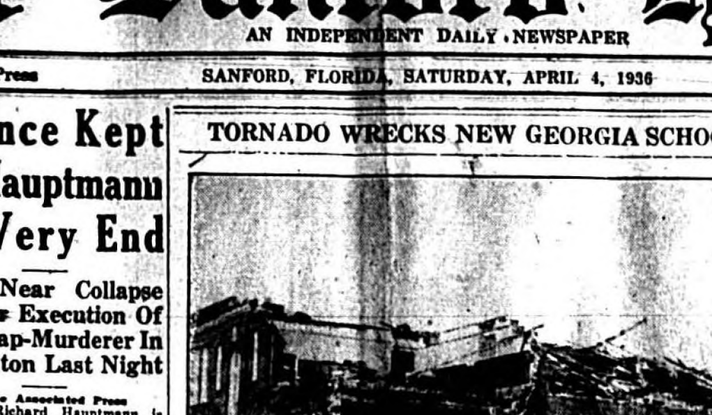
This new high school building was practically destroyed when a tornado ripped through Gordo, Ga., killing 16 persons and injuring 1,000. Hundreds of dwellings, among which were some of the city's finest, also were razed by the twister. (AP Photo)
