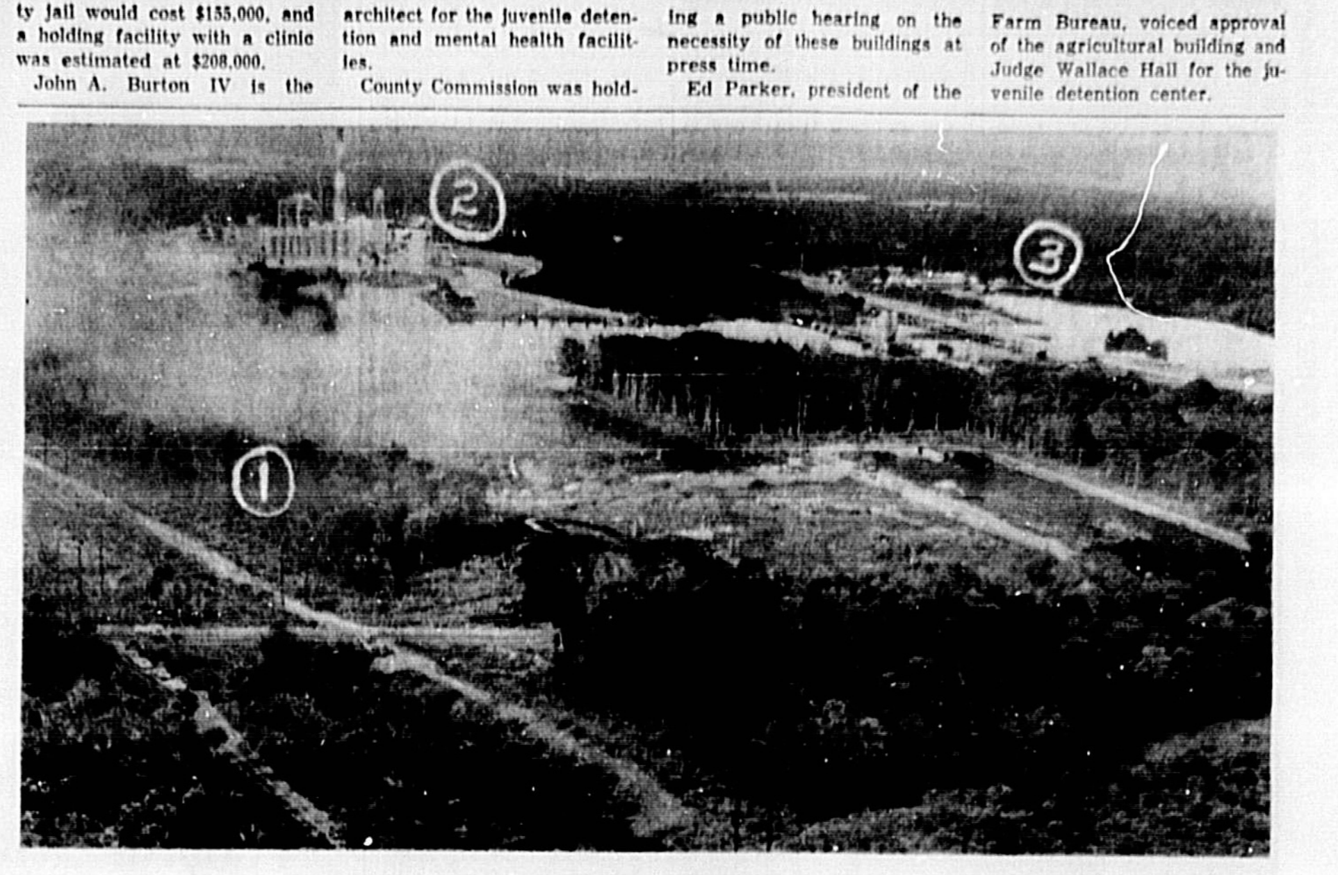
TOTE THAT BARGE . . . SANFORD PORT site from the air is pictured. Cleared area (center) will be occupied by the wharf and warehouse. Area covered by trees and smoke (No. 1) will be the barge basin, itself. Sixty-foot concrete pilings have been driven to test for footings for wharf and warehouse. Picture is looking east with Florida Power and Light Company (No. 2) and Lake Monroe Park and harbor (No. 3) just beyond the St. Johns River bridge.
