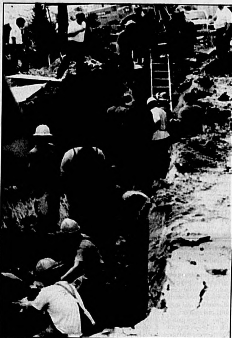
Emergency personnel respond to the scene of the cave-in. Two of the three men in the ditch at the time of the accident are reported to have been completely buried for at least five minutes.
